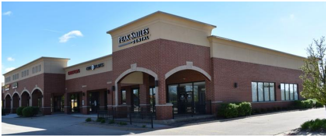
Above and Right – Phase I - Randall Crossing – Algonquin, IL One story 36,000 sq. ft. retail facility. The foundation system consisted of caissons and grade beams due to poor soil.
