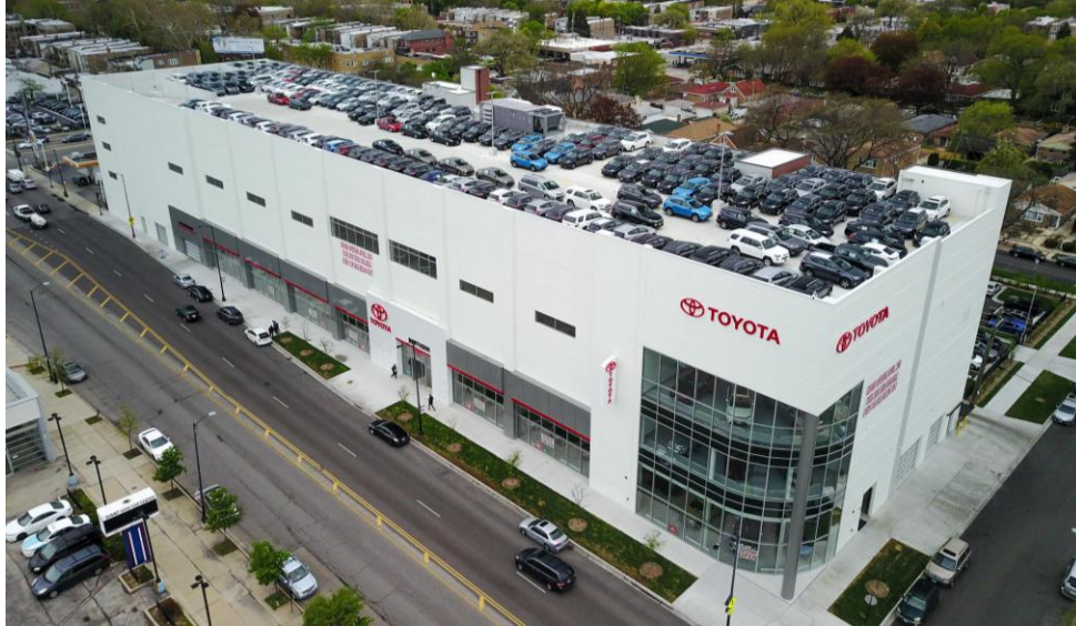
Northside Toyota Dealership 6060 N. Western Ave., Chicago, IL – New 4-Story Auto Dealership included sheet piling design for poor soil, caisson design and unique grade beam design for high torsional or twisting loads.
