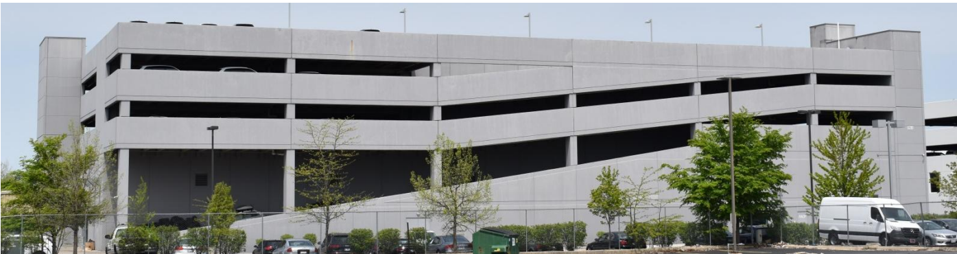
Audi Westmont Garage Car Storage and Auto Repair on Ground Level - Unique structural engineering design for parking garage includes a mix of caissons and shallow spread footings due to highly variable soil. The garage design is based on seismic forces governing over lateral wind forces.
