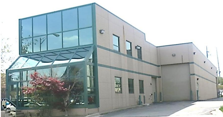
Above Left - Des Plaines Glass – Des Plaines, IL – Structural design of a new precast panel building. Incorporated into design of precast were overhead cranes running full length of building.
