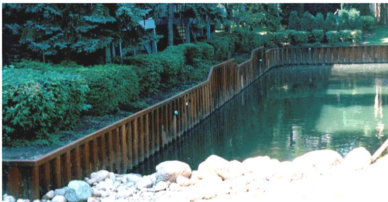
Left – Cantilever sheeting design and installation for retention of soil at pond at the Ancient Tree Condominium Complex in Northbrook, IL
