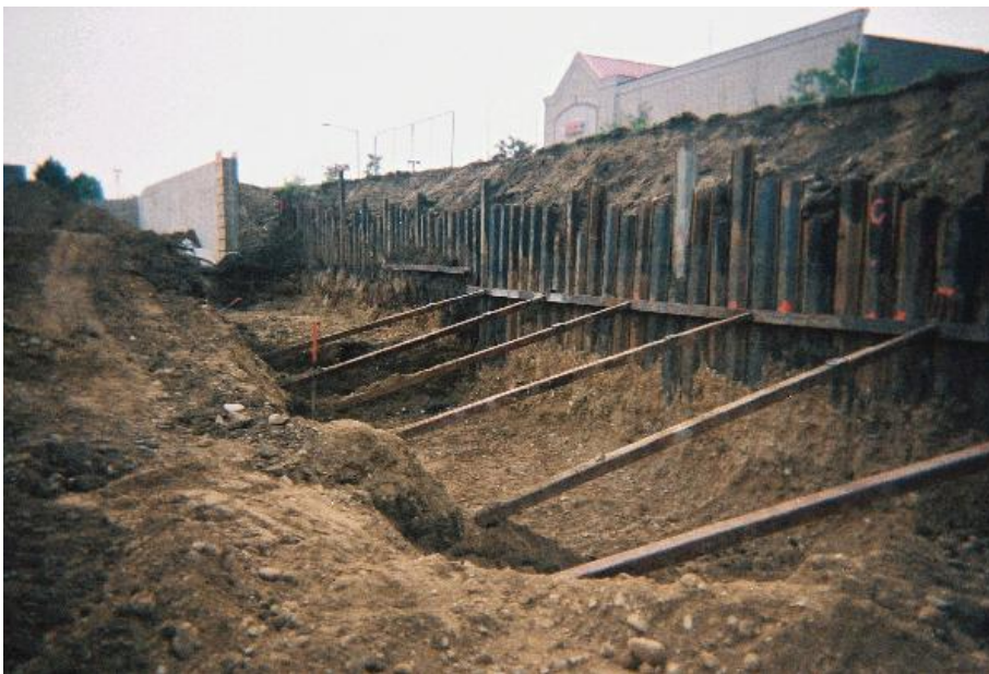
Left - Cary, IL - Earth retention system for Fienburg Court Roadway.
