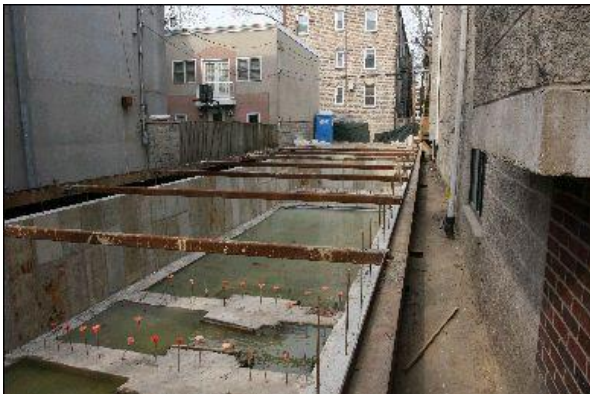
Left – Bracing for 4 story condominium on N. Fremont Avenue in Chicago.
