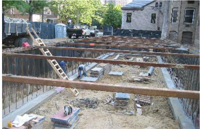
Typical braced sheeting system to achieve an excavation depth less than 12'-0" depth. Chicago, IL
