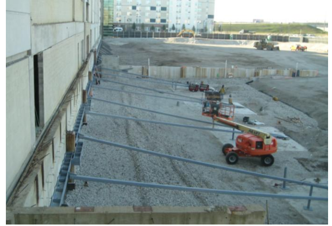
Above Left - Wall bracing to create resistance for lateral soil pressure at The Park in Rosemont. Diagonals shown resist tension forces. Above Right - Overview of wall bracing installed to resist forces from soil backfill at The Park in Rosemont.
