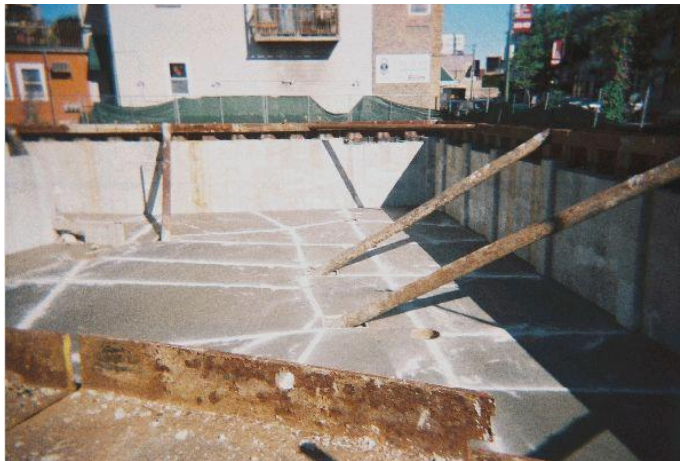
Above Left- North Milwaukee Avenue – Chicago. Earth retention system with an excavation depth greater than 12'-0" required Board of Underground review. Above Right – Chicago - Design based on Board of Underground criteria for a mat foundation. Included structural design for condominium and retail facility. Excavation depth was also greater than 12'-0" Board of Underground was required.
