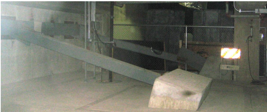
Above - Basement level wall bracing design for The Park in Rosemont. Thrust resistance from wall was designed using helical anchors grouping diagonally embedded in the soil.
