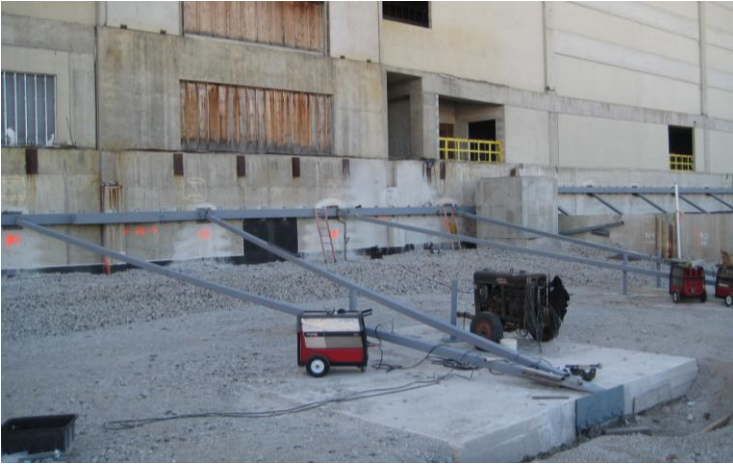
Above Left - Wall bracing to create resistance for lateral soil pressure at The Park in Rosemont. Diagonals shown resist tension forces. Above Right - Overview of wall bracing installed to resist forces from soil backfill at The Park in Rosemont.
