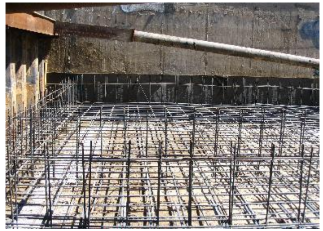
Above Left- North Milwaukee Avenue – Chicago. Earth retention system with an excavation depth greater than 12'-0" required Board of Underground review. Above Right – Chicago - Design based on Board of Underground criteria for a mat foundation. Included structural design for condominium and retail facility. Excavation depth was also greater than 12'-0" Board of Underground was required.
