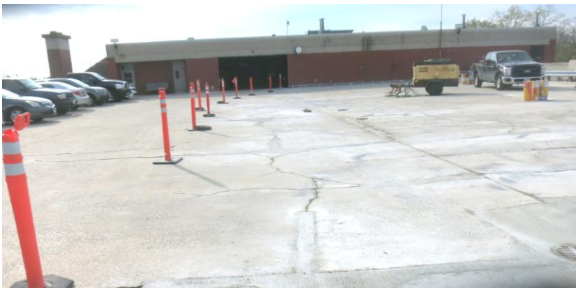
Left–Park Ridge, IL Maintenance Facility Restoration Repairs. Engineering analysis and investigation for development of repair documents for top deck concrete deck repair solutions and for masonry cracking of the Facility. Photo shows crack repair, underway for cracks up to 3” cracks.
