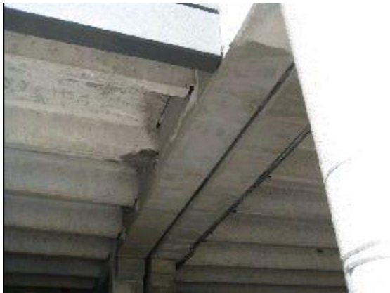
Beam repairs Completed
