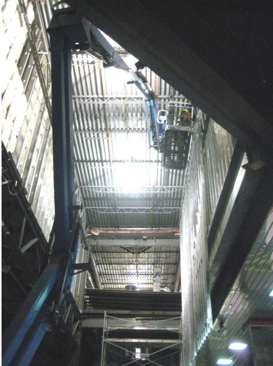
Left and Above - Rosemont Convention Center – New entrance to “G” Hall. Structural engineering design and construction services to add a new three-story atrium for entrance to second floor “G” Hall. Left is a birds-eye view of creation of new atrium
