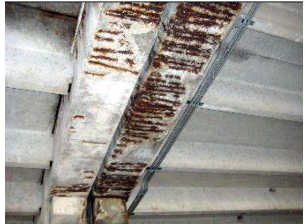
Beam Deterioration Before Repair
