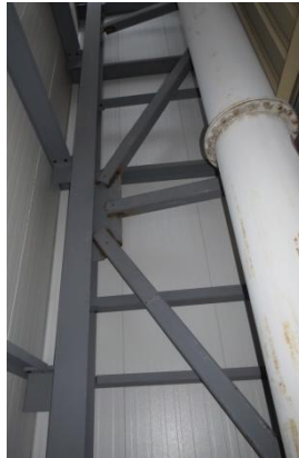
Wieland Metals – Wheaton, IL – USA – Above Left Photo – German manufacturing facility for precision steel expanding vertically. Construction underway shown in photo. Part of expansion included a ton crane runway shown above left using W36 girders. Above Middle - vertical bracing of the system shown. Above Photo Right – New processing line mat foundation. Helical Anchors used for new column placement while facility production continued without lapse or slowdown.
