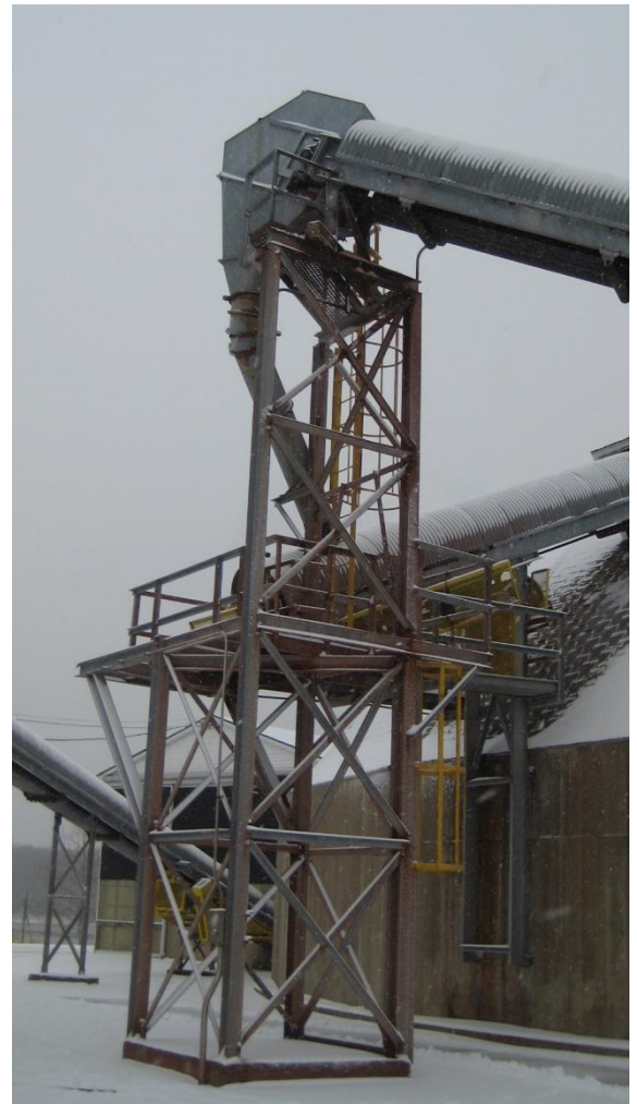
Above - Potash Manufacturing Facility – PCS / Phosphate Feed Ingredients Plant- Marseilles, IL – Structural analysis and investigation with repair documents for repairs to settlement and shifting of existing facility.
