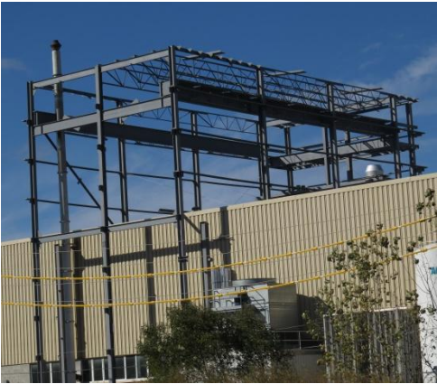
Wieland Metals – Wheaton, IL – USA – Above Left Photo – German manufacturing facility for precision steel expanding vertically. Construction underway shown in photo. Part of expansion included a ton crane runway shown above left using W36 girders. Above Middle - vertical bracing of the system shown. Above Photo Right – New processing line mat foundation. Helical Anchors used for new column placement while facility production continued without lapse or slowdown.
