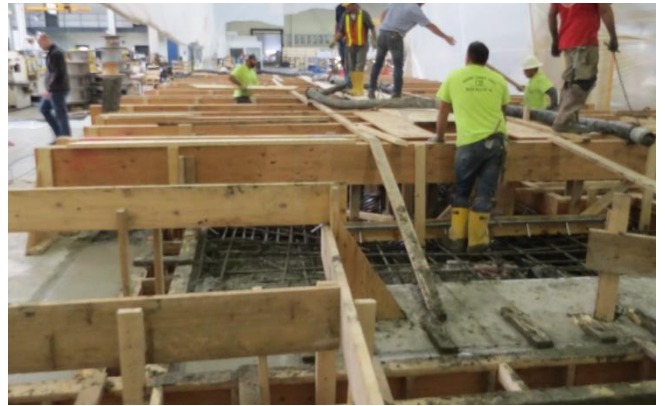
Wieland Metals – Wheaton, IL – USA – Above Left Photo – German manufacturing facility for precision steel expanding vertically. Construction underway shown in photo. Part of expansion included a ton crane runway shown above left using W36 girders. Above Middle - vertical bracing of the system shown. Above Photo Right – New processing line mat foundation. Helical Anchors used for new column placement while facility production continued without lapse or slowdown.
