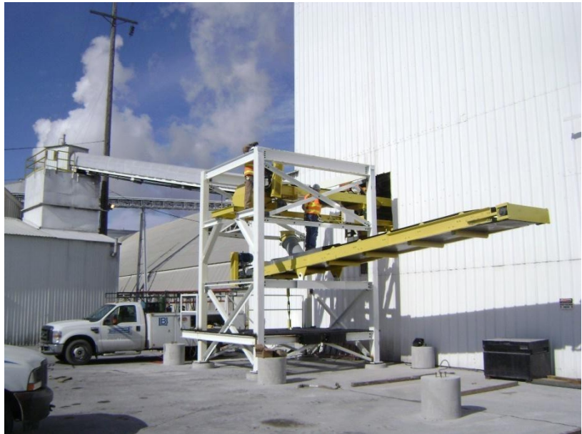
Above Left – Potash Shipping Building – PCS / Phosphate – Marseilles, IL – Structural engineering investigation and analysis for the installation of a new conveyor and unloading system assembly into an existing pallet shipping building. Above Right - PCS/Phosphate – Marseilles, IL – Design and documents for container Loading System at Shipping Area.
