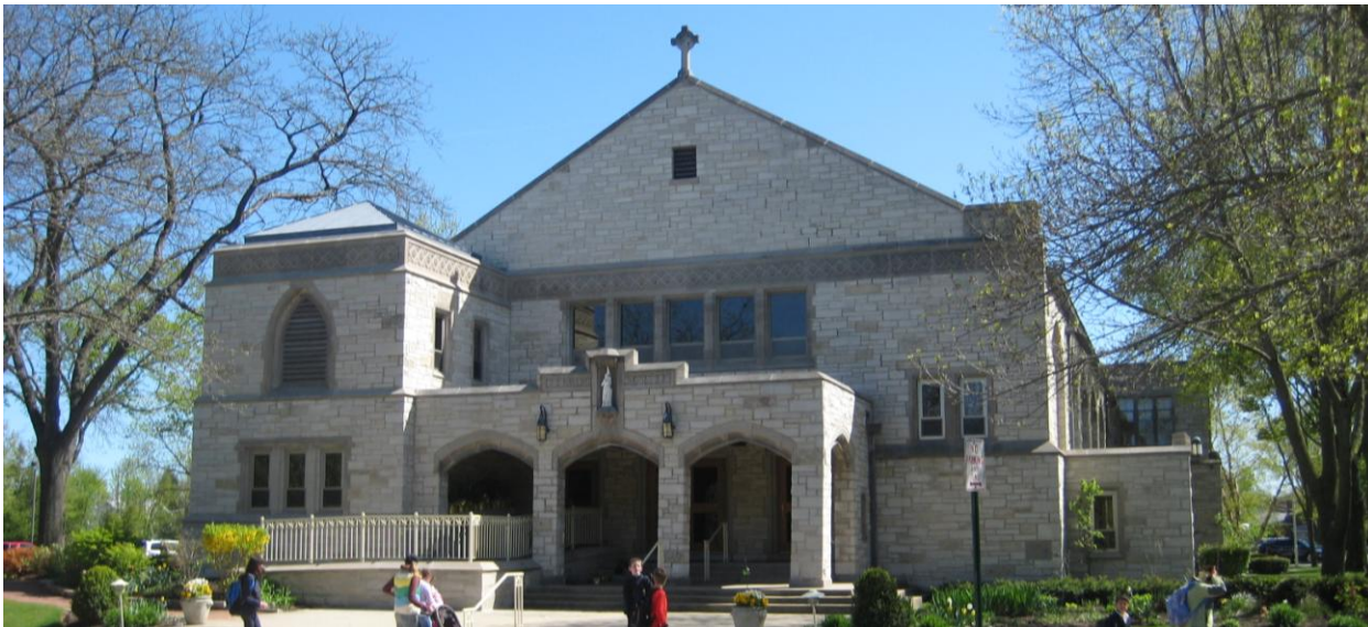
Above - St. Joan of Arc – Skokie, IL – Structural replacement of main church canopy entrance. New steel framing installed and existing limestone reinstalled. Damaged limestone matched and replaced with new limestone.
