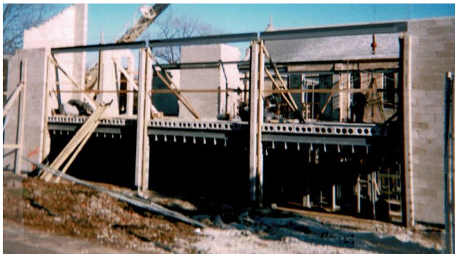
Above – All Saints Cathedral – Polish National Church – Chicago, IL. Photos above show completed church addition and work under construction. Structural design included steel framing, masonry bearing walls and precast concrete.
