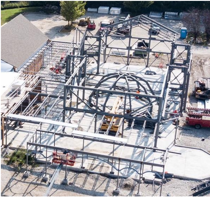
Above Left – Drone photo of a new Greek Orthodox Cathedral we designed shows framing with dome to be installed. Dome was lifted into place later with four tower cranes.
