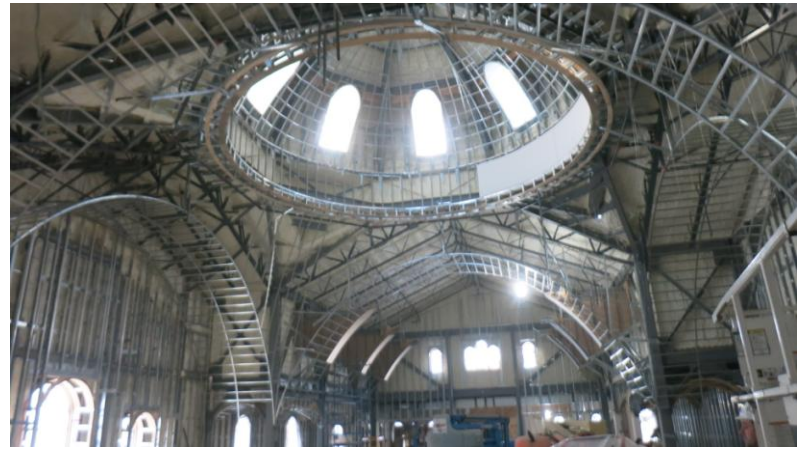
Above Left – Drone photo of a new Greek Orthodox Cathedral we designed shows framing with dome to be installed. Dome was lifted into place later with four tower cranes.
