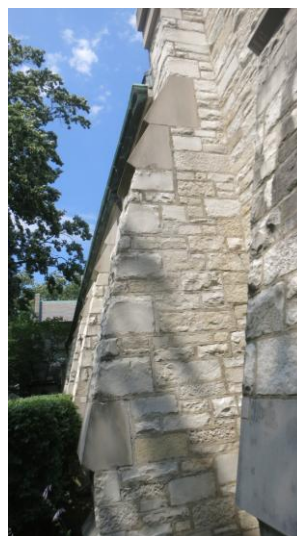
Far Left – St. Francis Xavier Catholic Church- Wilmette, IL. – Structural investigation of Gothic church constructed in 1939 to ascertain the cause of cracking of buttresses supporting the roof.
