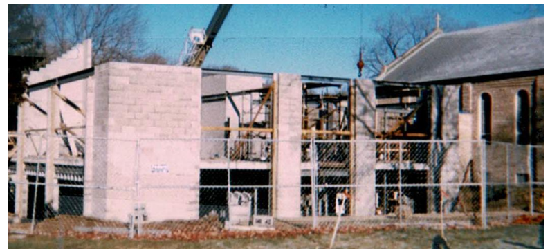
Above – All Saints Cathedral – Polish National Church – Chicago, IL. Photos above show completed church addition and work under construction. Structural design included steel framing, masonry bearing walls and precast concrete.
