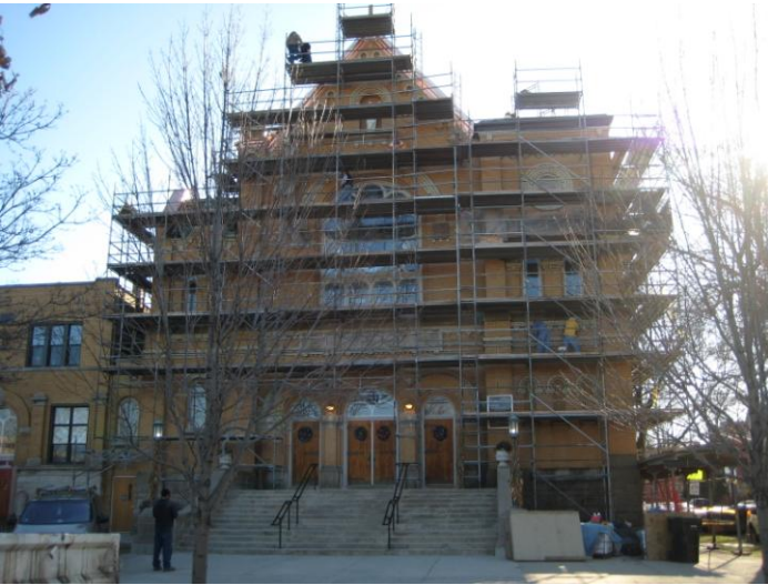
Above - St. John Berchmans Catholic Church – Chicago, IL – Five year structural repair program to the parish campus included restoration of church, administrative building and schools (5-building campus). Repairs included replacement of steel framing due to deterioration, bell tower framing repairs, roof truss system repairs and replacement with steel trusses in the main church and masonry repairs on all buildings.
