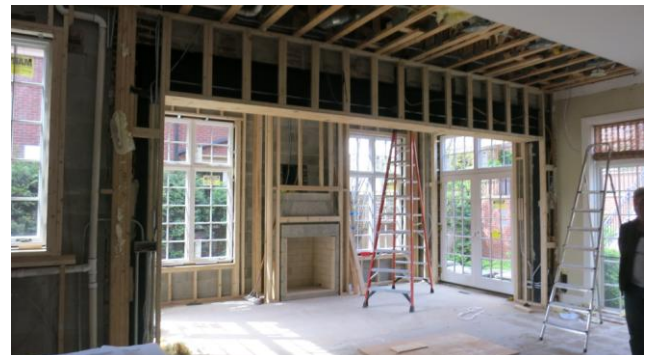
Mohawk Avenue Chicago, IL – Structural engineering for new 1 story addition with basement shown above. Two story bearing wall required the design of a shoring system to remove a bearing wall and create a new open space.
